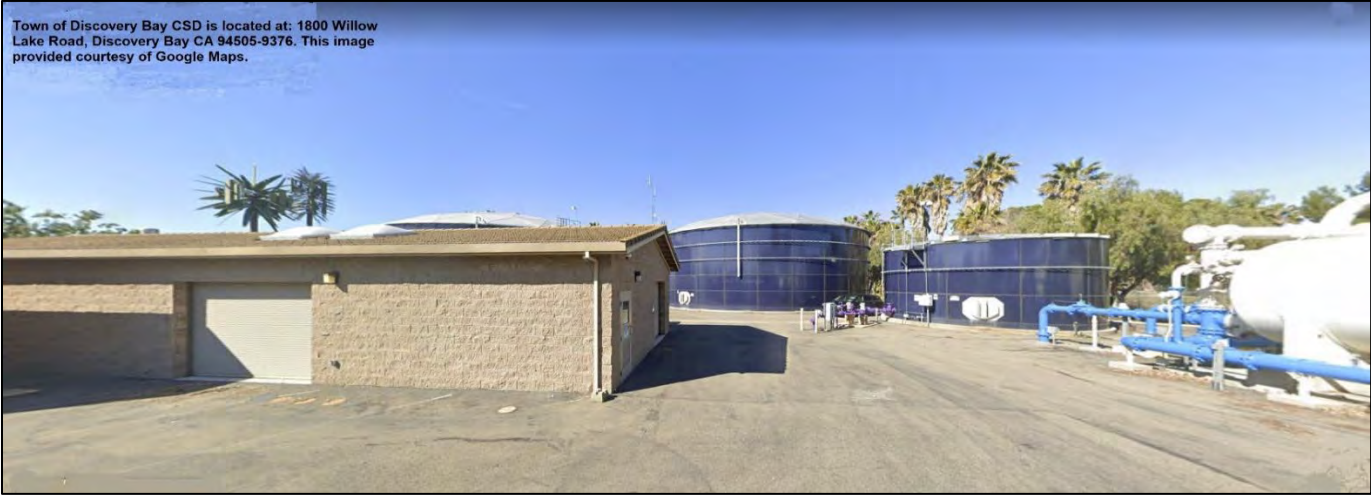
Figure 21-2: Street View of TODBCSD Facilities
