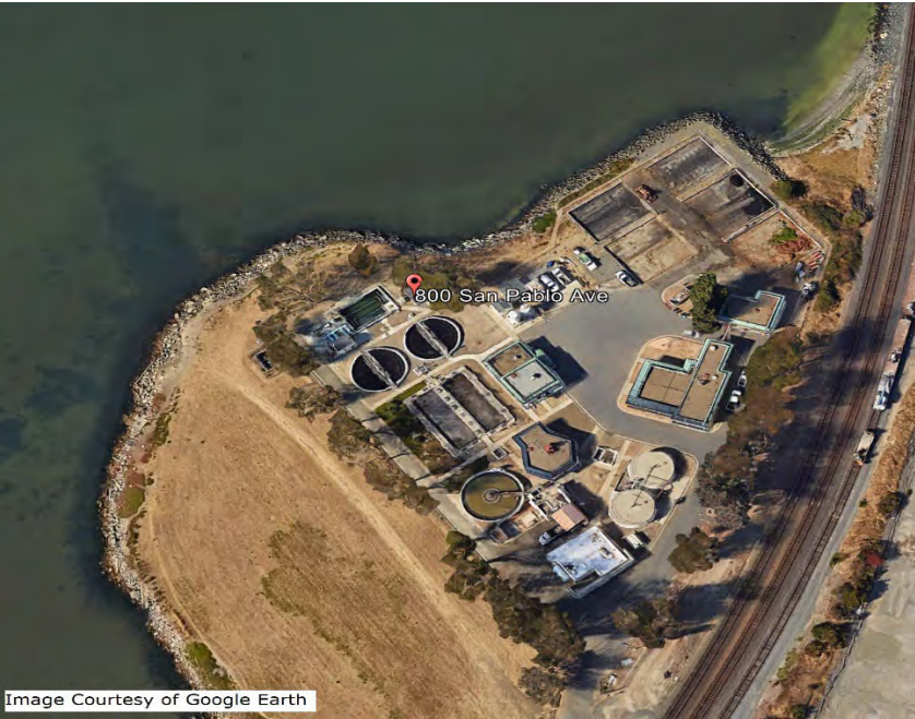
Figure 19-4. View of the Rodeo Sanitary District Facilities
