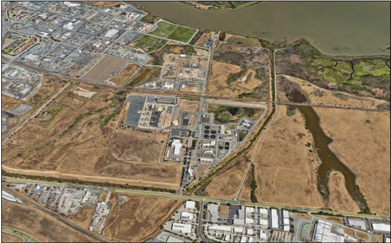
Aerial Image of Wastewater Treatment Plant located in Antioch. Image courtesy of Google Earth
