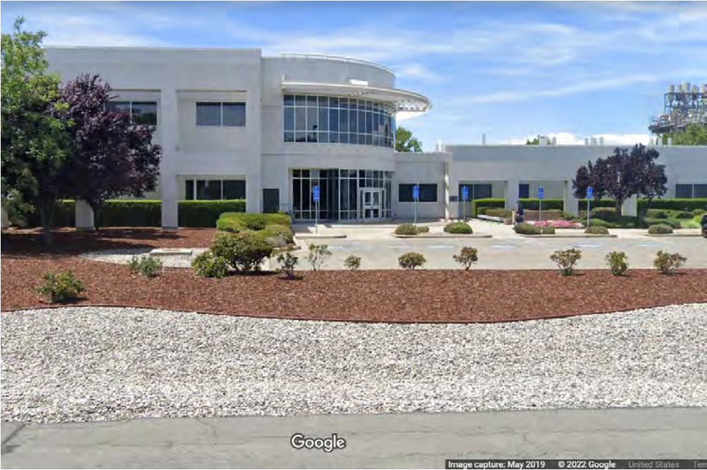
Figure 14-2: Google Maps Street View of the Delta Diablo Plant Operations Center
