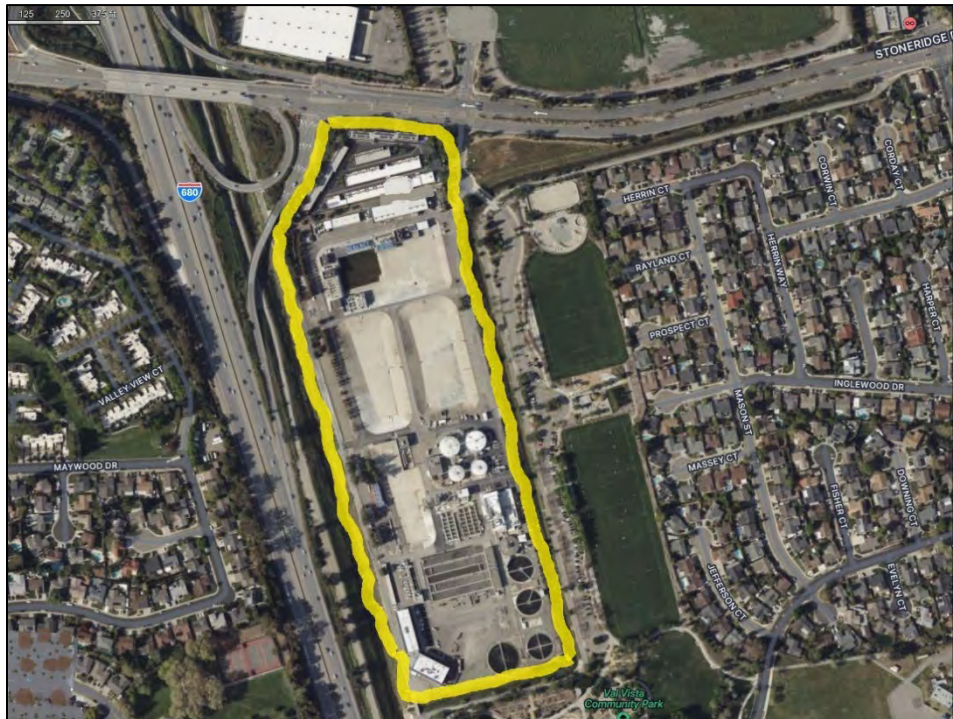
Figure 15-2: Satellite View of Wastewater Treatment Facilities at 7399 Johnson Drive in Pleasanton
