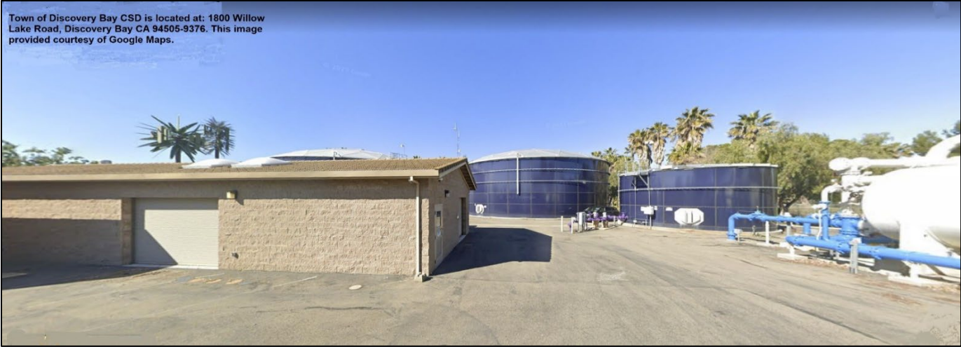
Figure 21-2: Street View of TODBCSD Facilities
