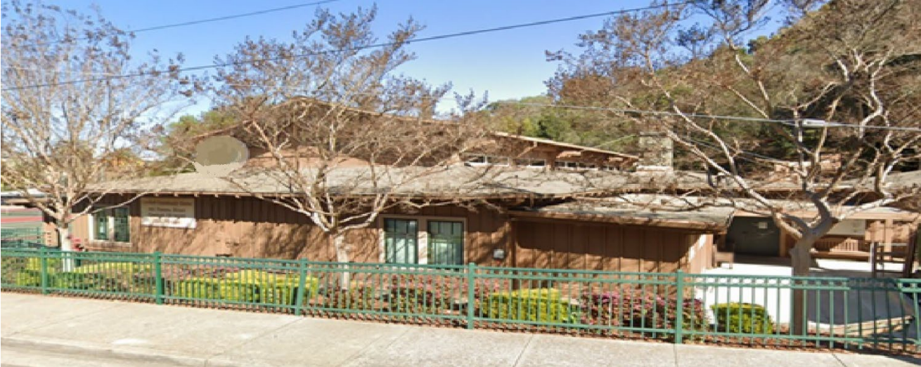
Figure 13-3. Google Maps Street View of the Crockett Community Center
