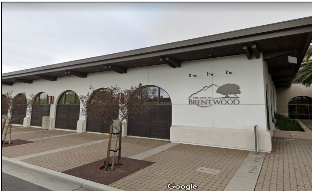
Figure 4-2. Google Maps Street View of the Brentwood City Hall
