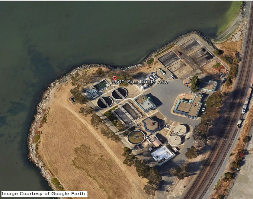
Figure 19-4. View of the Rodeo Sanitary District Facilities
