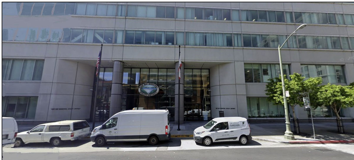
Figure 16-2: EBMUD Administration, 375 11th Street, Oakland, CA 94607-4240 Courtesy of Google Maps
