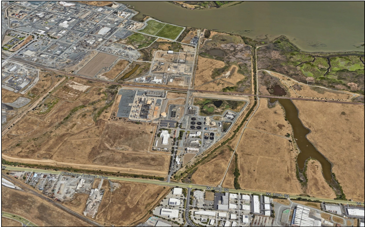
Aerial Image of Wastewater Treatment Plant located in Antioch. Image courtesy of Google Earth
